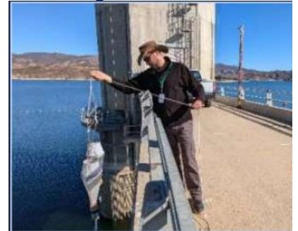
Veliger sampling at Castaic Lake – MWD January 13, 2025
