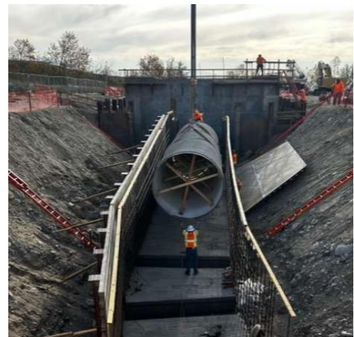
96-inch diameter pipe installation for Inland Feeder-Rialto Pipeline Intertie. MWD January 22, 2025
